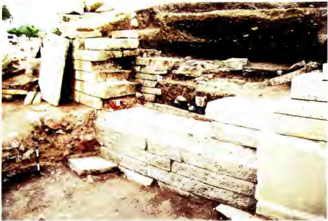
A. Inner veneering of the core, south-east of Mahā Stūpa
