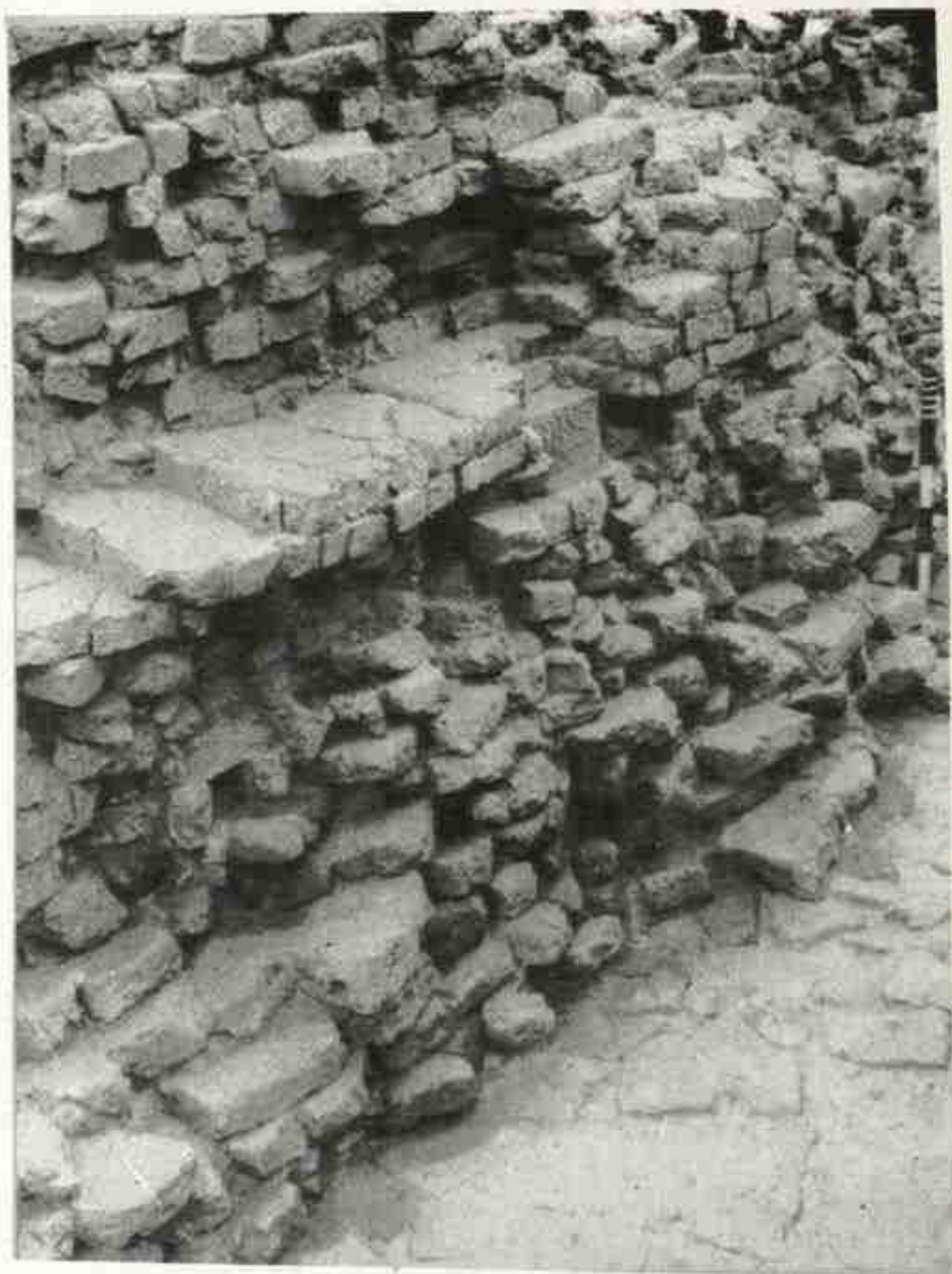
A view of the eastern side-wall of the Inlet Channel. The broken stone in the centre seems to have been a part of the slab over which the incoming water used to pass. Looking east. See pp. 23 and 48
