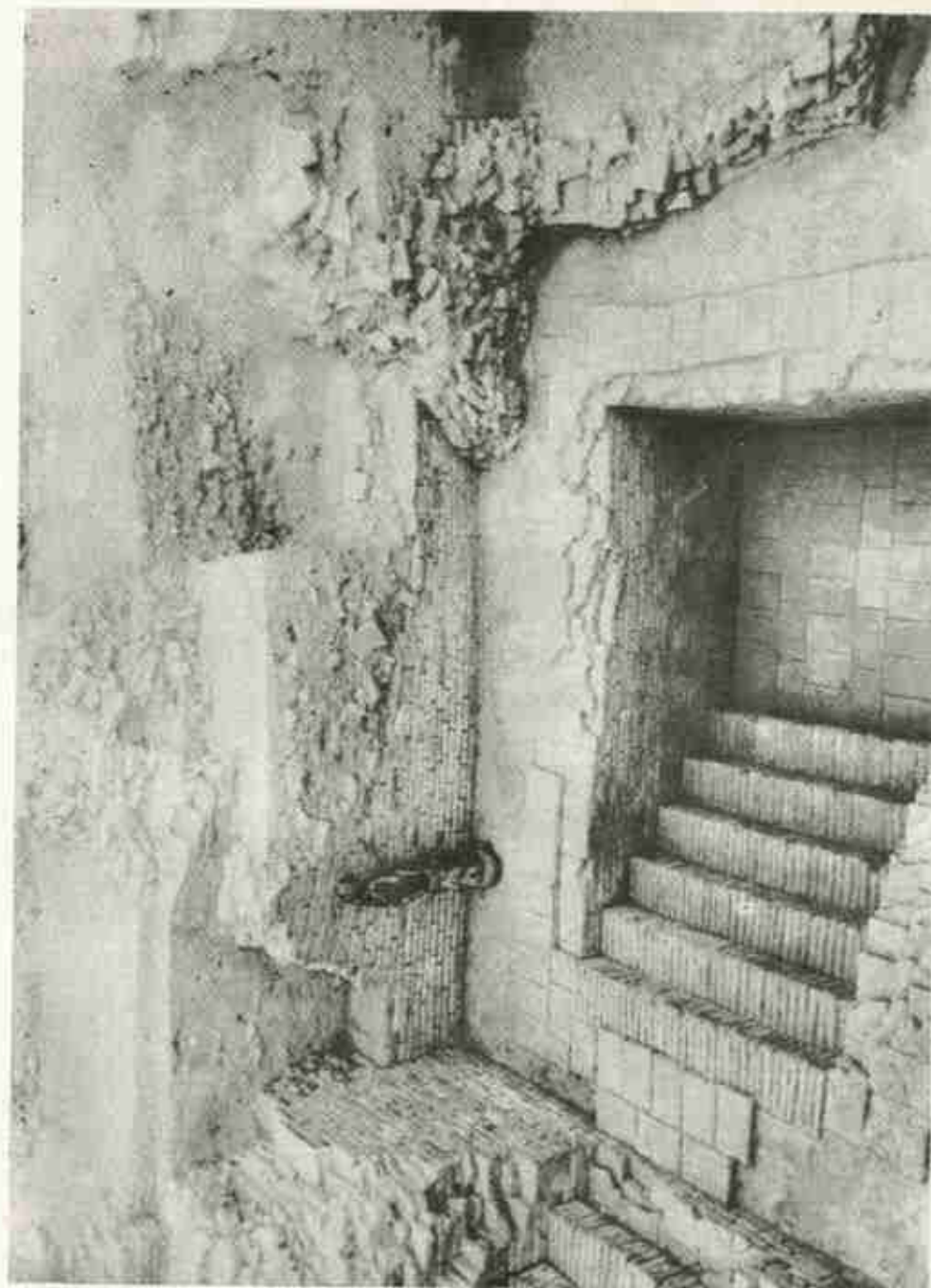
A part of the staircase with badly damaged Second and Third Retaining Walls in background. Looking east. See p. 33
