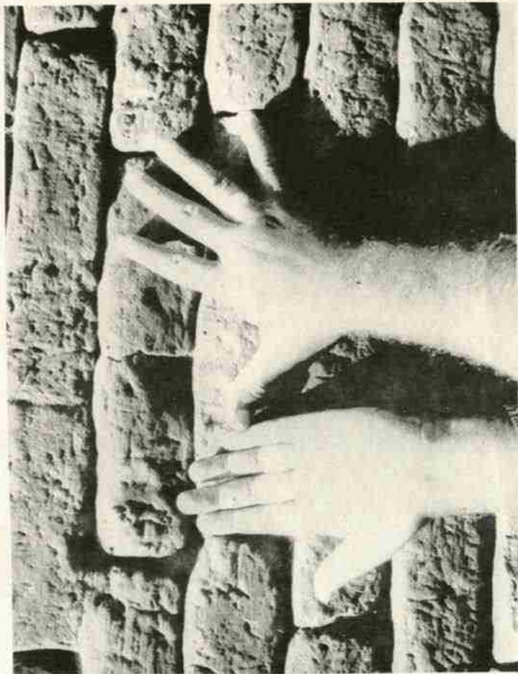
Close-up of a part of the Lowest Retaining Wall on the eastern side of Tank A. The bricks measured one vitasti (span) and four angulas (finger-widths) in length. See p. 43
